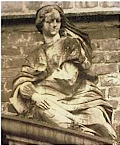
Fig. 1. Time-lapse photos of statues at Herten Castle near Recklinghausen, Westfalia, Germany, built in 1702. The left side picture was taken in 1908, the right side picture 1969, showing almost complete destruction of the surface. Porous Baumberg sandstone is composed of mostly quartz grains which are cemented with soluble calcite. Photos and information were supplied by Mr. Schmidt-Thomsen, Landesdenkmalamt Westfalia-Lippe, Münster, Germany.
