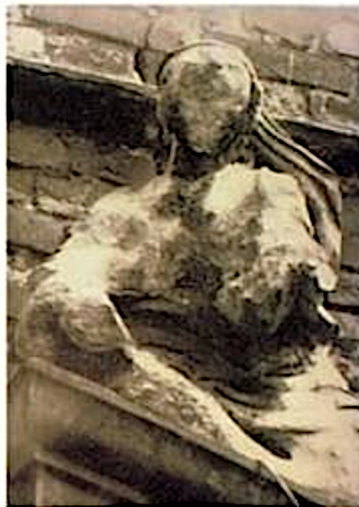
Fig. 1. Time-lapse photos of statues at Herten Castle near Recklinghausen, Westfalia, Germany, built in 1702. The left side picture was taken in 1908, the right side picture 1969, showing almost complete destruction of the surface. Porous Baumberg sandstone is composed of mostly quartz grains which are cemented with soluble calcite. Photos and information were supplied by Mr. Schmidt-Thomsen, Landesdenkmalamt Westfalia-Lippe, Münster, Germany.
